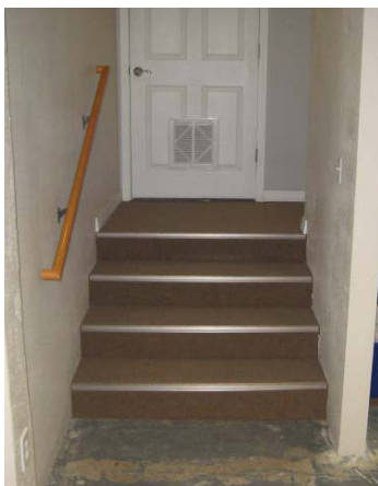
Image 7: Stairs within Primary Route
