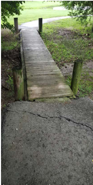
Image 50: Walking Trail Bridge
