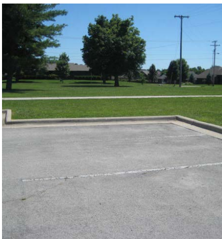
Image 53: Parking without Curb Cuts
