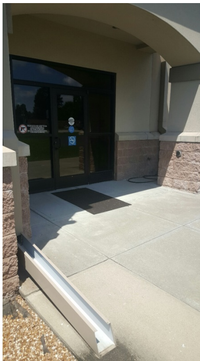
Image 17: Entry to Fire Station 1
