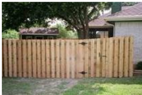
Typical Rear Yard Fence
